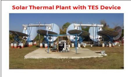
• System Design, Erection, Testing & Commissioning of 40 kWth and 10 kWe pilot plant aiming at the Feasibility Study of MWe Scale Concentrated Solar Thermal Plant integrated with 24 x 7 Thermal Energy Storage.
